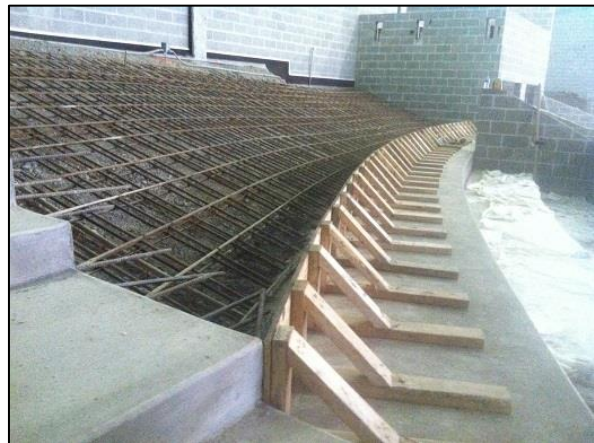
Figure 5: Auditorium Risers (Property of Mascaro Construction)
