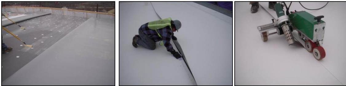
Figure 66: CWNCHS TPO Installation (Florida Consulting Property)
