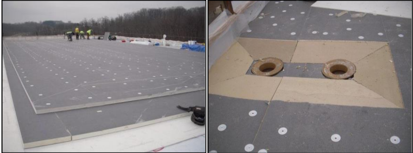
Figure 65: CWNCHS TPO Installation (Florida Consulting Property)
