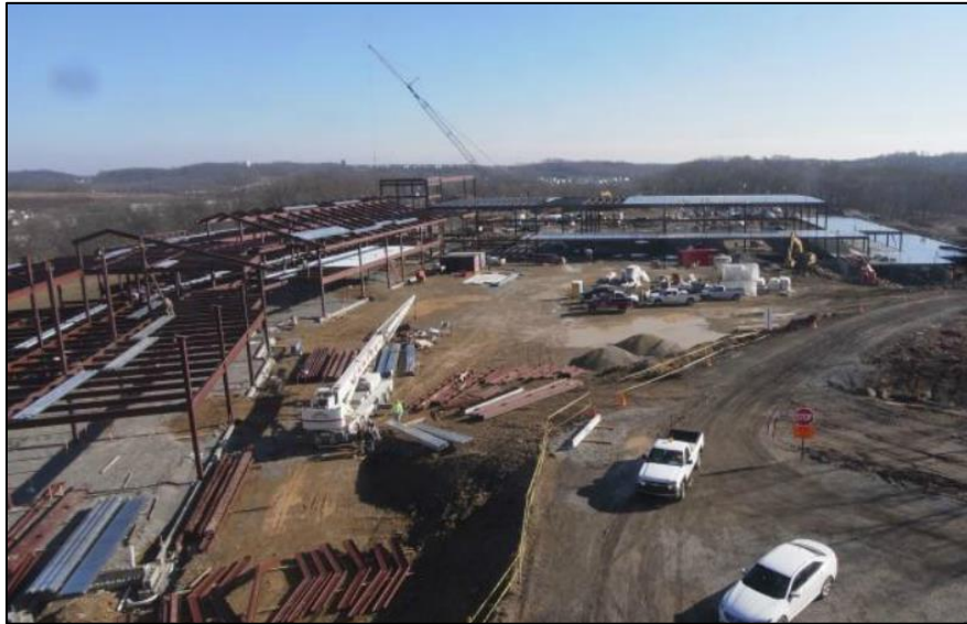
Figure 4: Steel Erection Phase (Property of Mascaro Construction)
