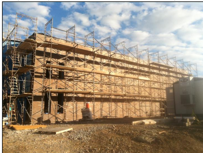
Figure 8: Brick Masonry Construction on Area E East (Mascaro Property)
